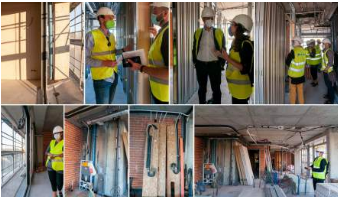
Figure 28. CASAIS session - Visit to a construction site
