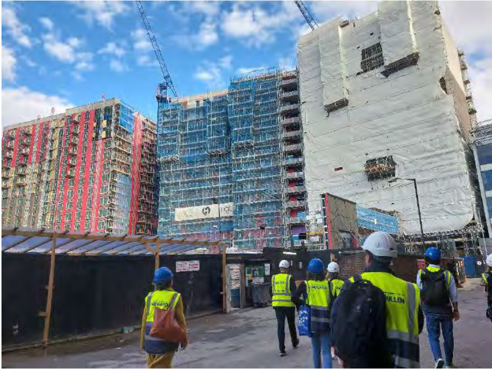
Figure 48. Group visit to construction site
